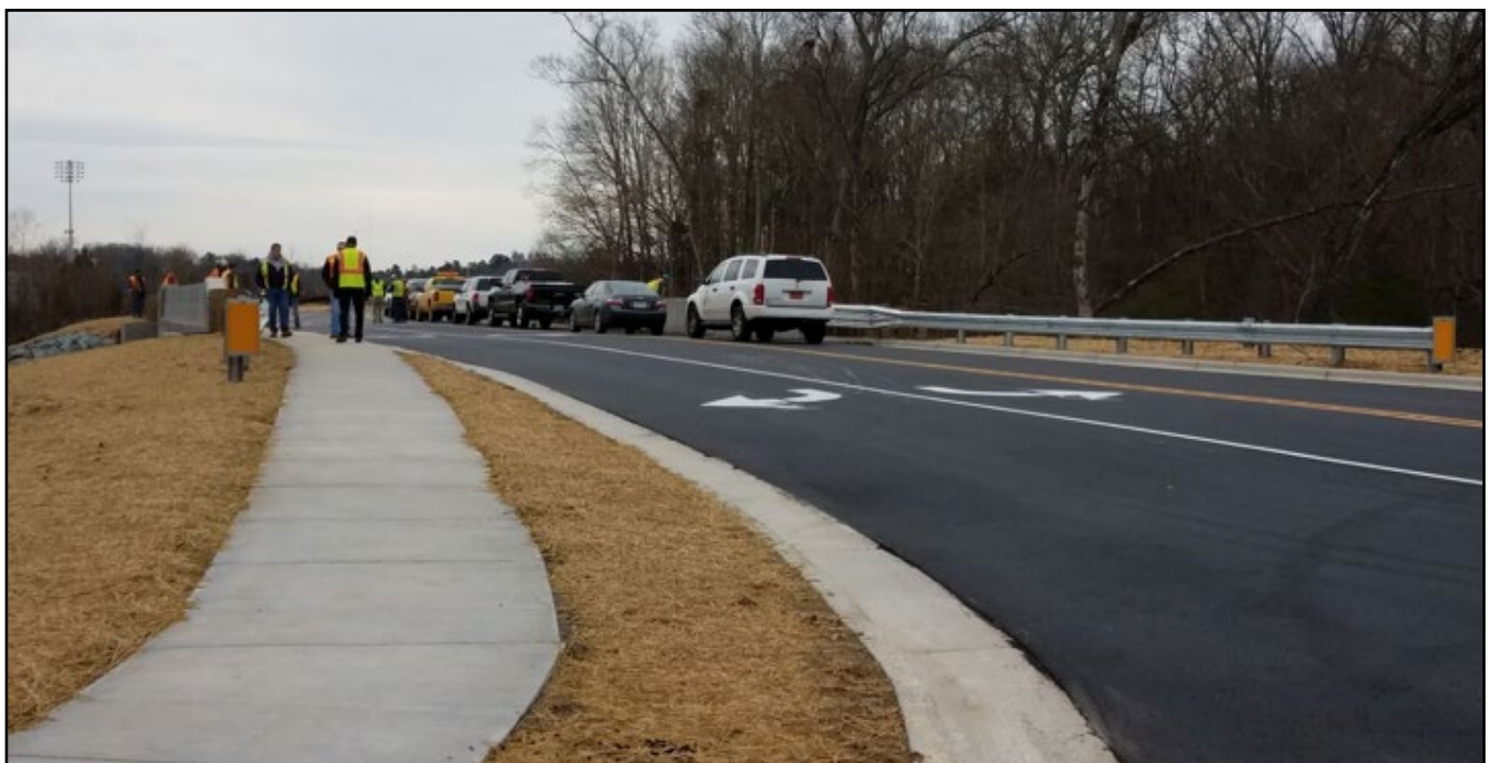
Bridge replacement project with new sidewalk - Raging Ridge Road at Stallings Road in Harrisburg.
